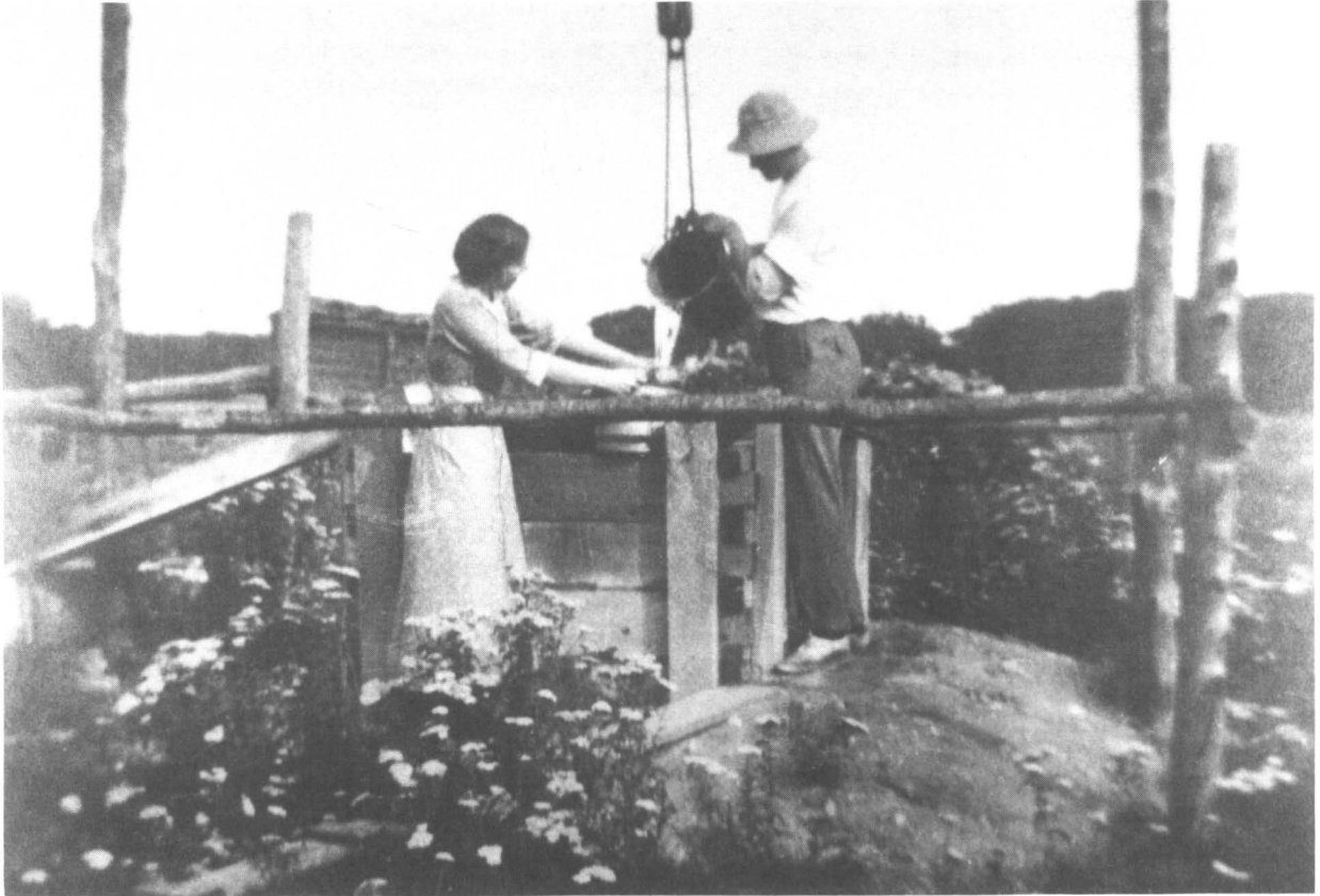
Authors' sister, Gale, and cousin, George, drawing water from sixty-foot-deep open well, in 1909. Dug by hand about 1865, the sides were shored-up with hand-hewn timbers
