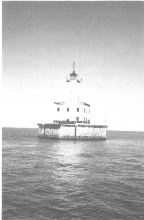
The "Crib"--a shoal warning-light near the Manitou Passage
