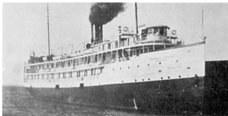
The puritan was built in Toledo for Graham and Morton Transportation Company in 1901. She was 257 feet long by 41 feet in the beam, powered by a 1500 horsepower engine. She was sold to N.T.C. in 1912. The Isle Royal Transit Company purchased the Puritan in 1933 and renamed it the George M Cox. She was wrecked on a pre-season voyage to Isle Royale, on a reef near Isle Royale, Lake Superior.
