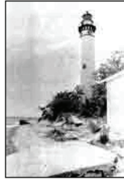
Erosion threatened the South Manitou lighthouse in 1986.
