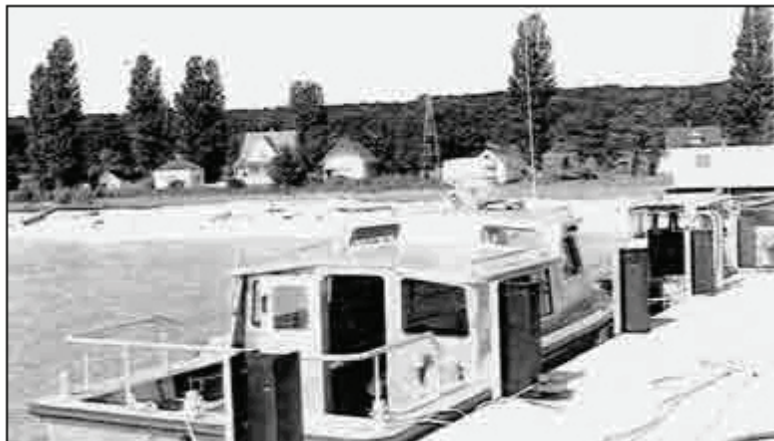
The newly constructed National Park Service dock at North Manitou Island, 1988.
