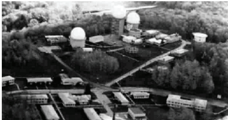
Former Air Force Base at Empire, adapted for use as a maintenance facility, c. 1987.
