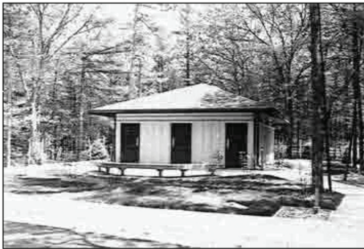
Modern comfort station at the expanded and improved Platte River campground, 1992.
