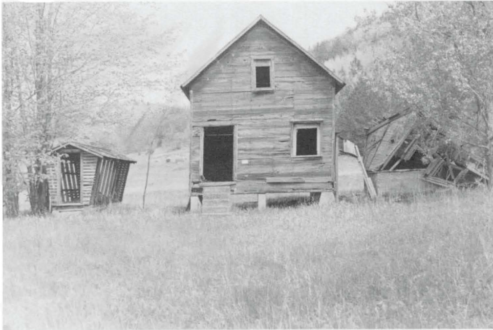
Figure 33. Farm buildings on Martin Basch farm, Port Oneida, 1993.
